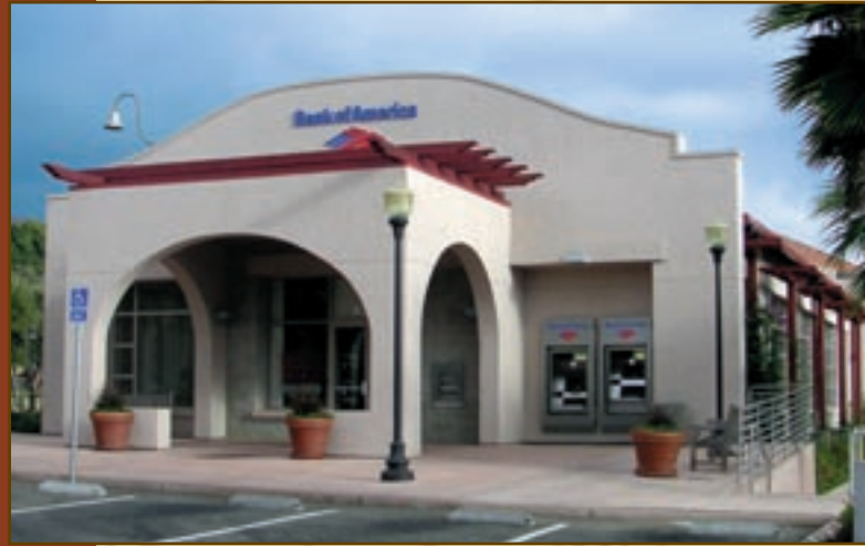
◀ New building, site and tenant improvement. —Mission San Jose, CA
