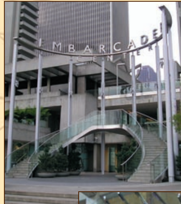
◀ New identity, staircase and canopy replacement project. —San Francisco, CA
