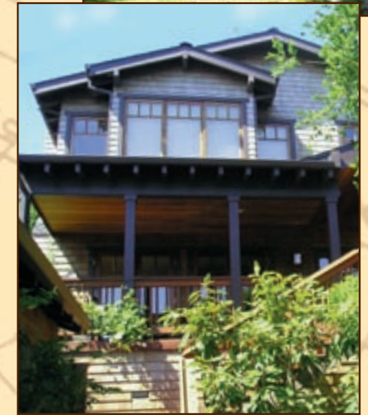
▲ New Construction of a craftsman style home. —San Rafael, CA
